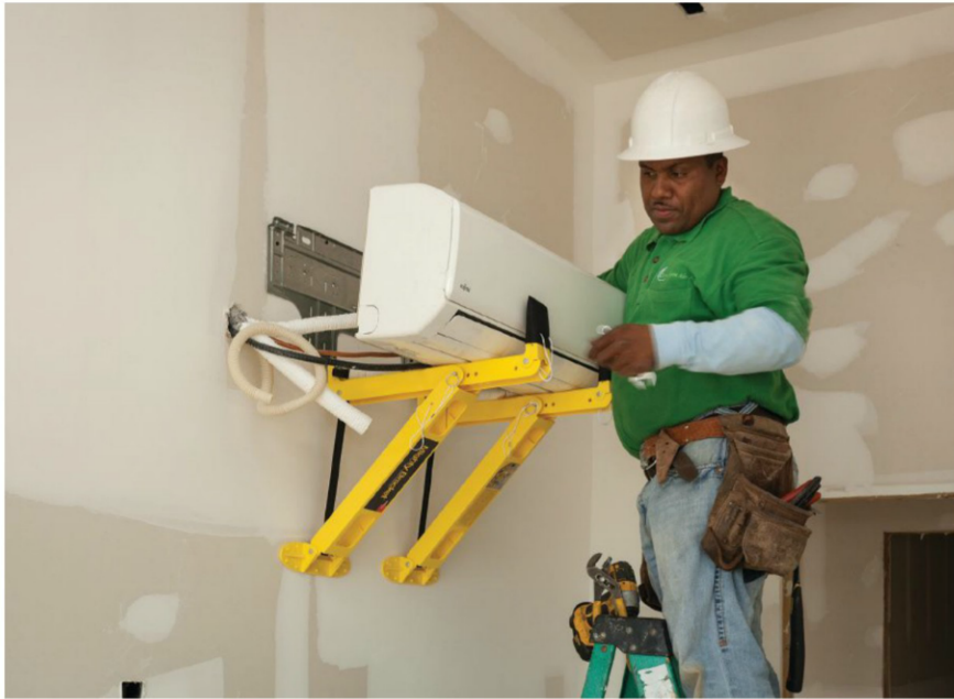
CUSTOM COMFORT: Chatham Pointe bedrooms feature high ceilings and are conditioned with small, wall-hung evaporators.
