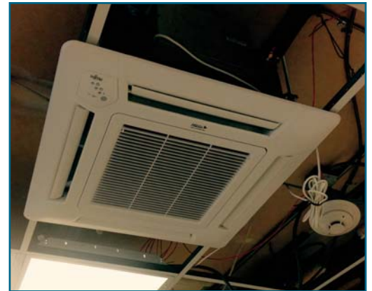
Shown is a compact cassette which is recessed into the ceiling, showing only the grille.
