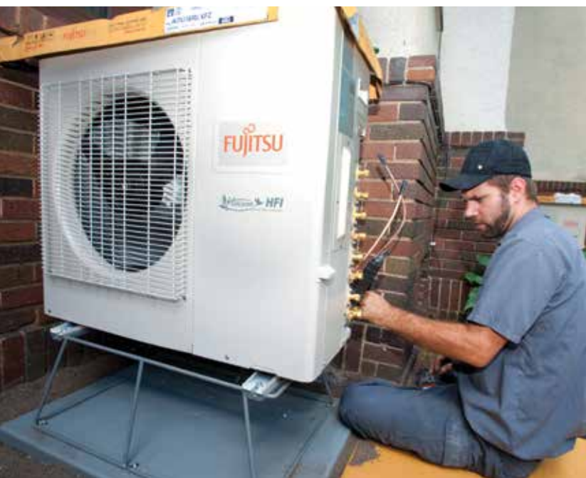
Andert makes a flare connection on the Rouner’s Fujitsu multi-zone condensing unit.
