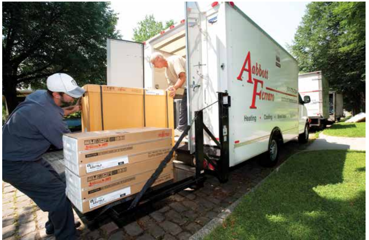
Philip Andert, project foreman, Aabott Ferraro, and Dennis Narog, installer, pull Fujitsu equipment from the truck for installation at the Rouner’s home. (Feature photos courtesy of Joe Szurszewski)
